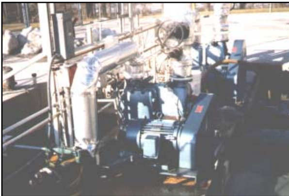
🔦 Megator H400 pumping paper mill backwater
