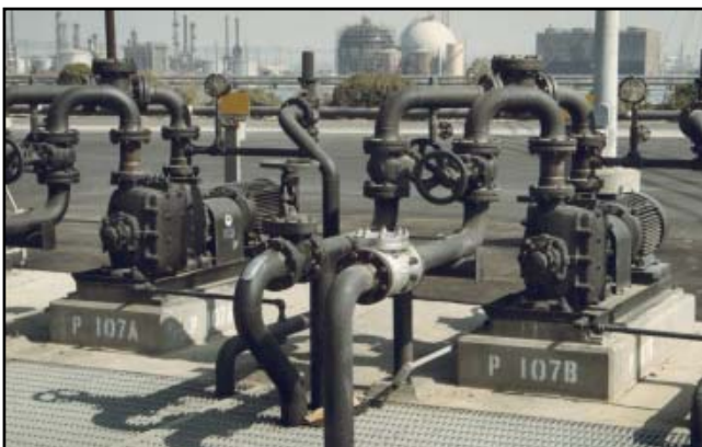
🔦 Two L400 pumps, pumping waste-water at an oil refinery
