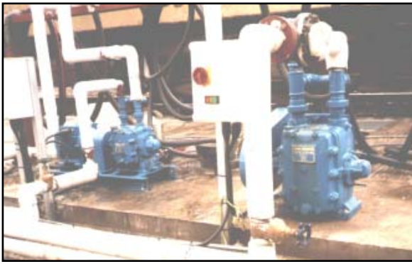
🔦 Pumping diesel fuel to a railway locomotive
