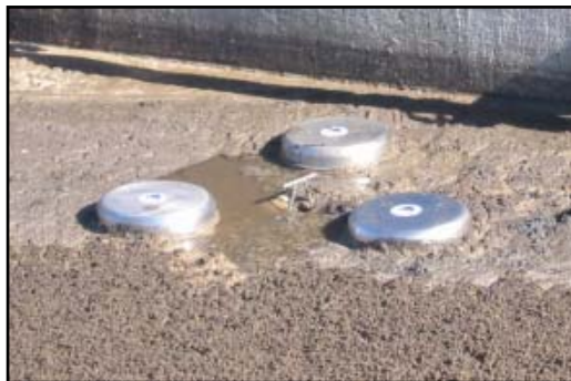
➤ Sewage scum removal
