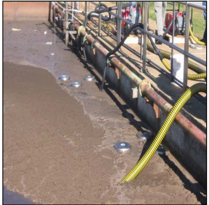
➤ Sewage tank during skimming cycle
