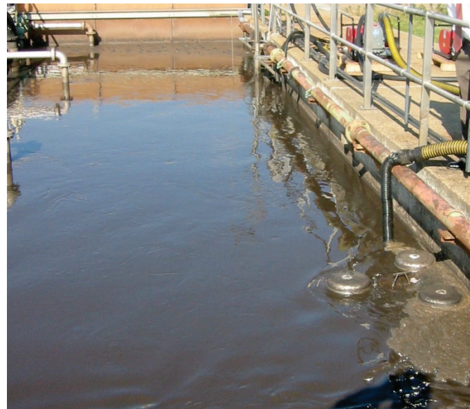
▲ Sewage tank after skimming cycle
