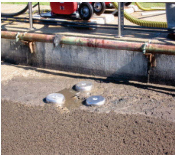
▲ Sewage tank before skimming cycle
